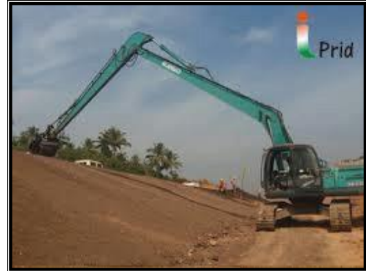
Fig-E3: Working of Slope Vibratory Roller
