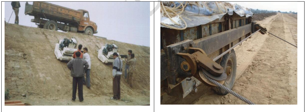
Fig-E1: Slope Compactor Working with counter balance Method
