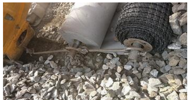
Fig-10.3(b): Linking of Rolls to BCM
