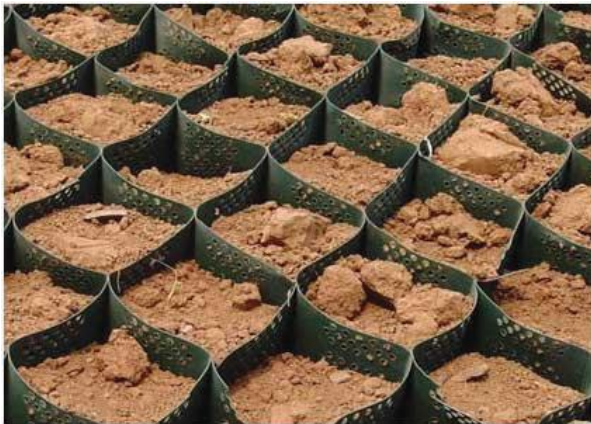
Fig-2.6(b): Geocell and it's applications
