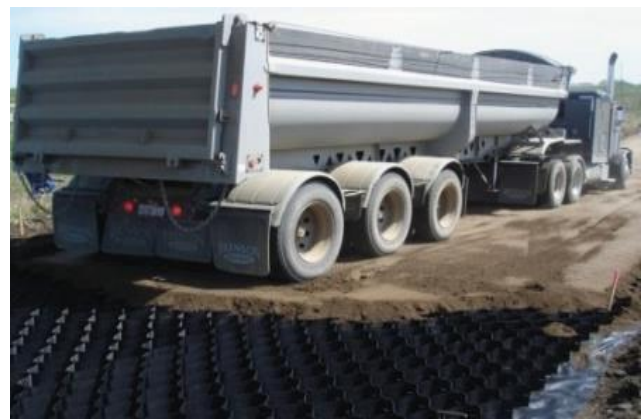
Fig-2.6(b): Geocell and it's applications
