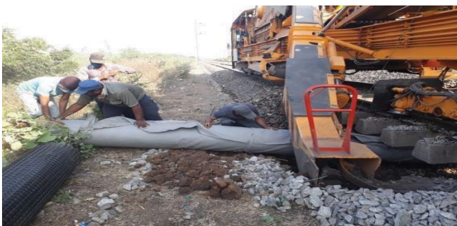
Fig-10.3(a): Insertion of Material under BCM
