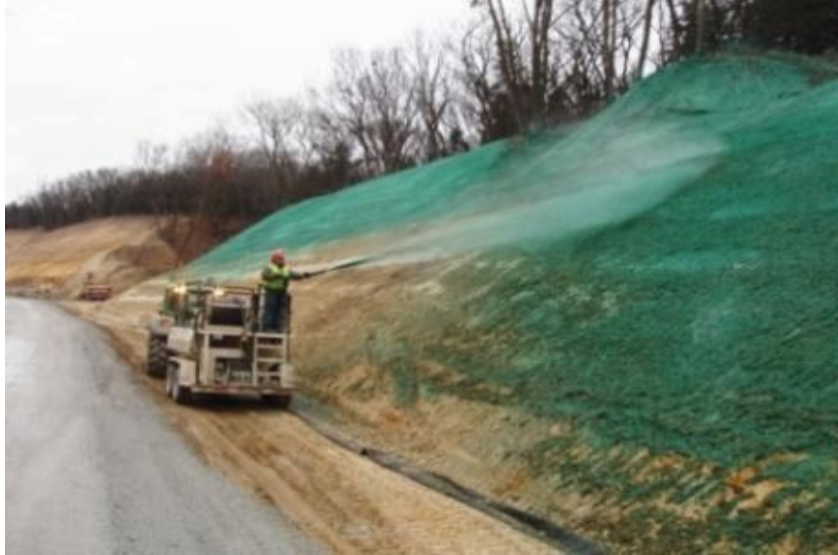
Fig-8.5 Figure showing Hydro-seeding/hydro-mulching on slope
