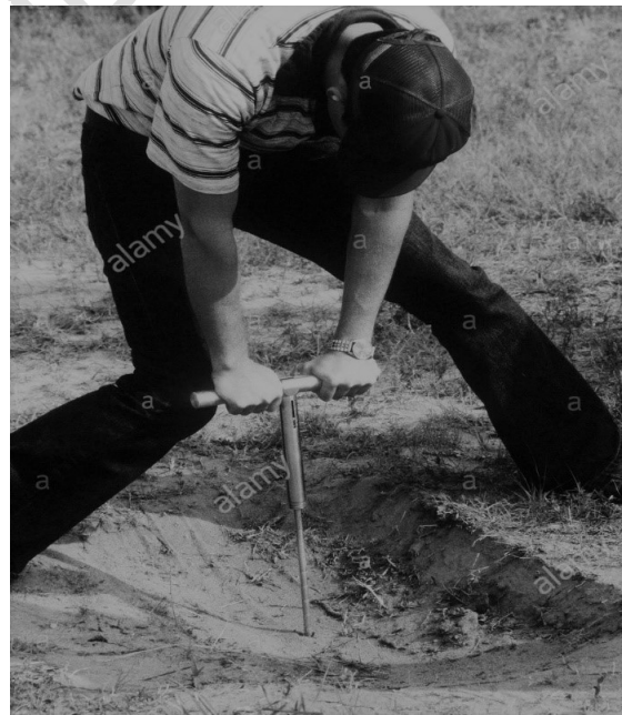
Figure 3: Standard Penetration Test (SPT)
