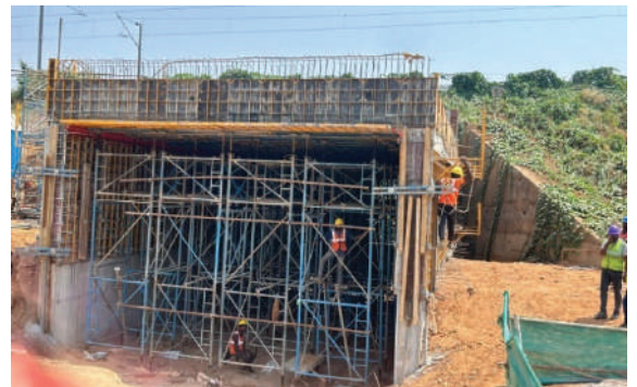
MIB-405 Top slab pouring completed between station of Myderahalli-Shettyhalli
