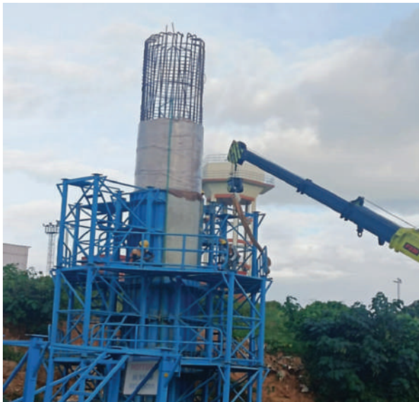
UP216 pier at YPR
