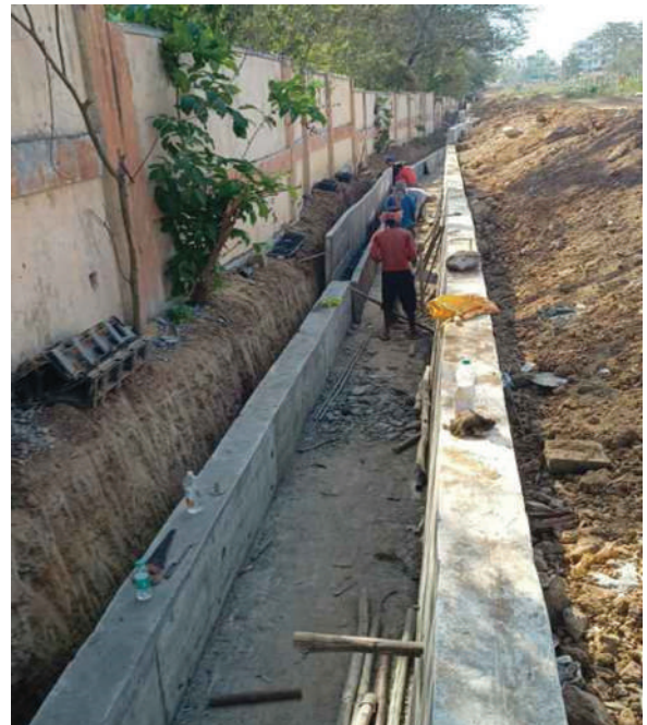
Retaining wall Cum Drain work
