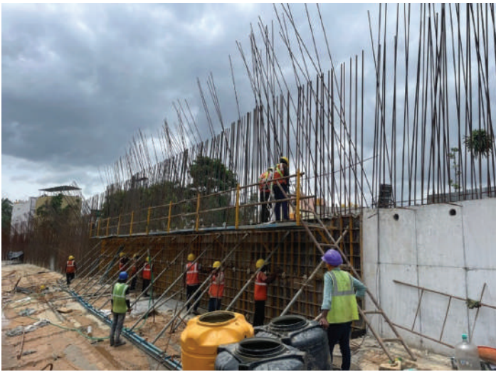
ERS work at kanaka Nagar
