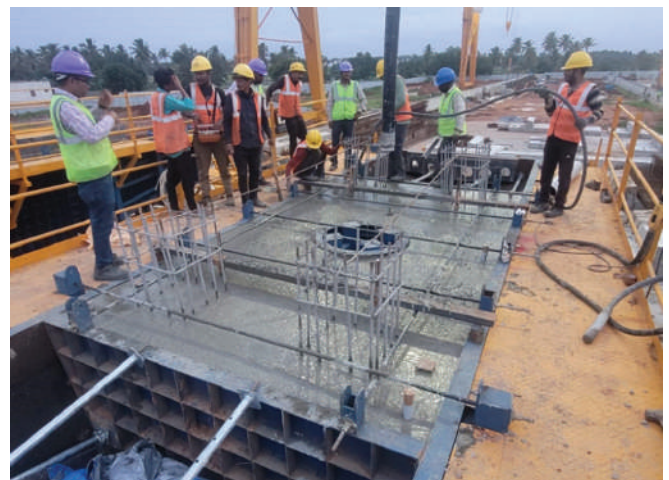
Precast Pier Cap in progress
