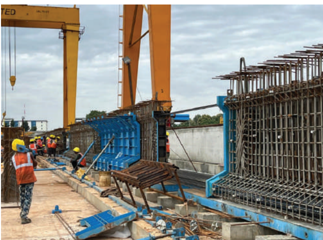
I girder work in progress
