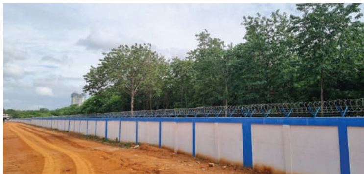
533-meter-long Air force boundary wall work at Jalahalli
