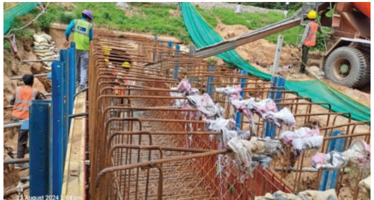
Bottom raft concreting progress for MIB -526
