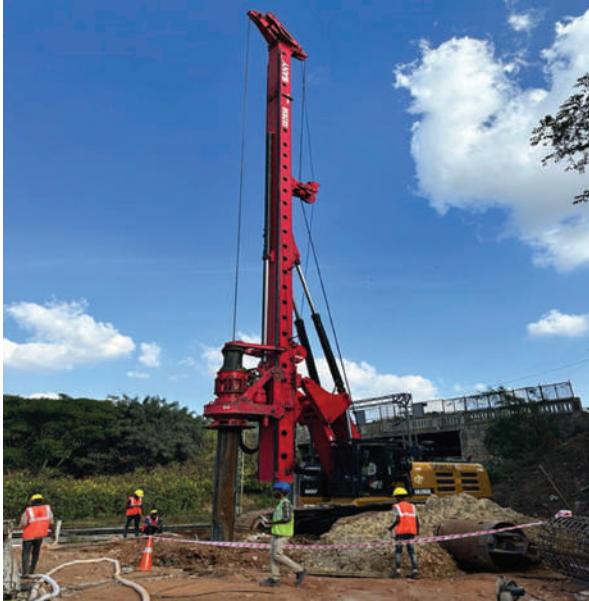
BH-177 (ROB 408B) test pile bore in progress
