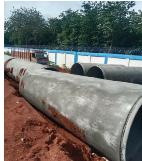
BWSSB: Diversion in progress
