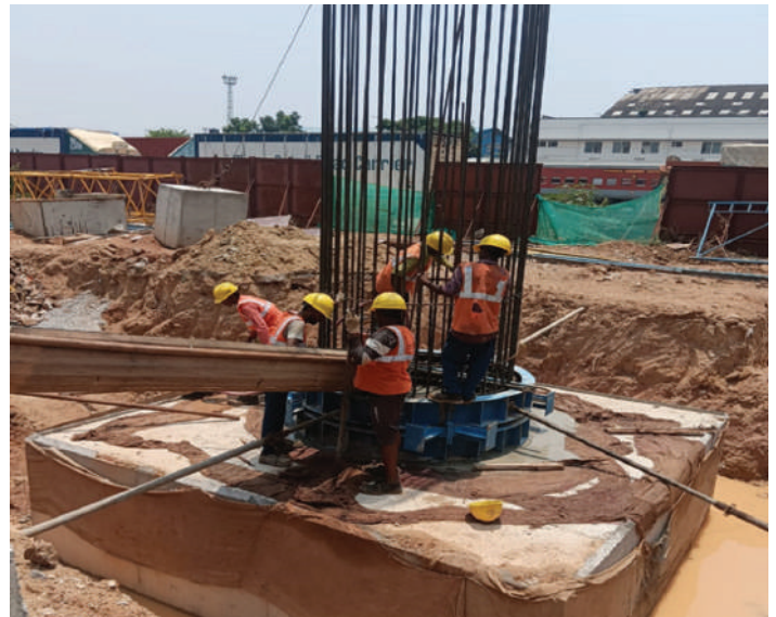
YPR UP208 Pier starter concrete
