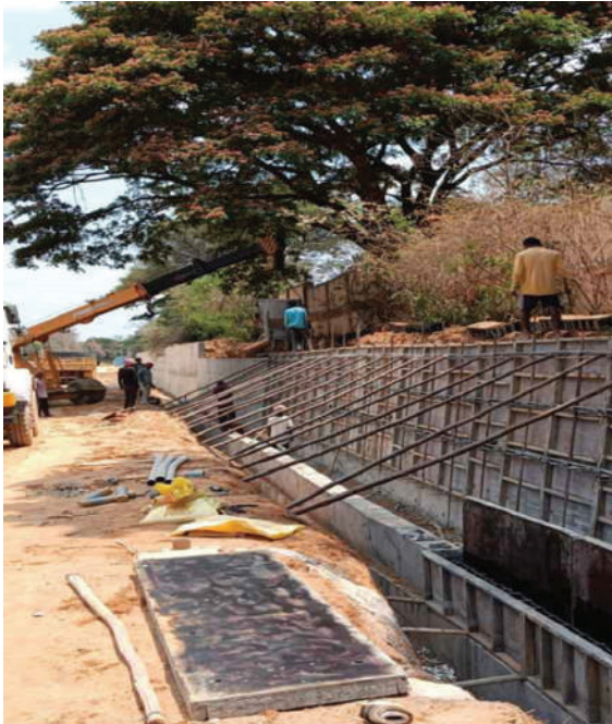
Retaining wall at Ch 206/950
