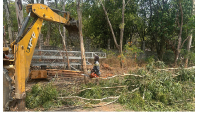
Tree cutting work is in progress at Heelalige station
