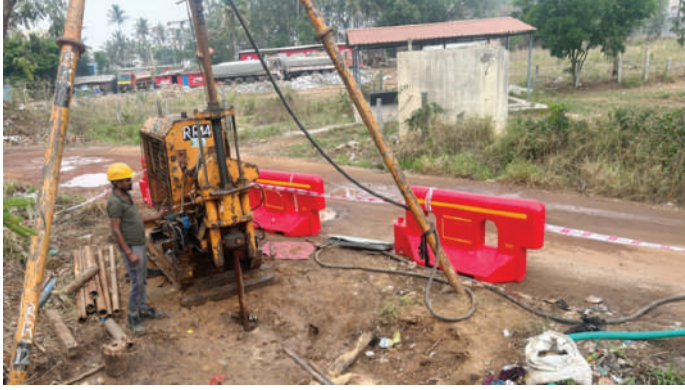
GTI work is in progress
