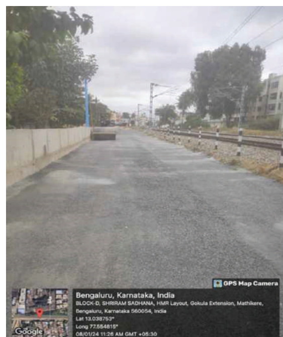
Blanketing work at Ch. 221/200
