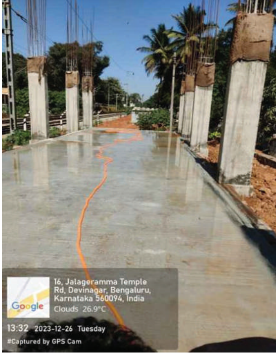
Lottegollahalli station Building work at YPR – Hebbal
