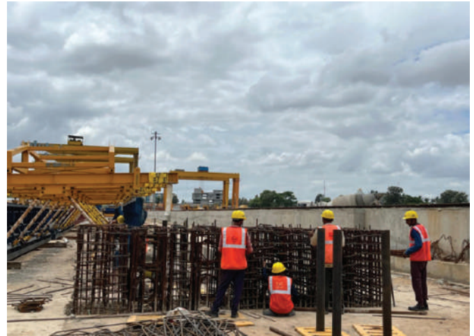
Gollahalli casting yard: U -girder bed line no-2 stressing end thrust wall reinforcement tying work
