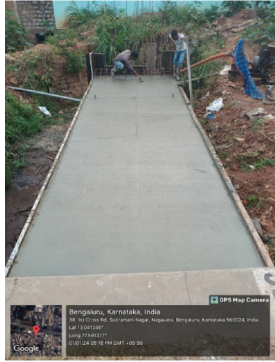
Minor bridge no 566 Top slab. Concrete work (YPR-HEB Block section)
