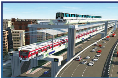
Shared alignment (common Right of way) between BMRC & BSRP at Benniganahalli (500m)
