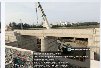
Bridge 412 PSC Slab Launching
