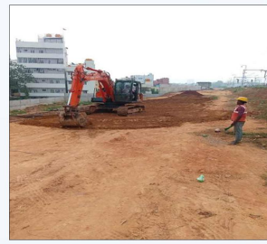
Formation Soil Levelling Works at Yesvantpur Yard
