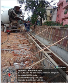
Retaining Wall Concrete works Near Mathikere
