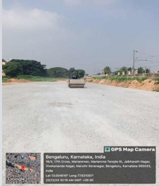
Blanketing Layer Compaction Works Near Banaswadi Yard
