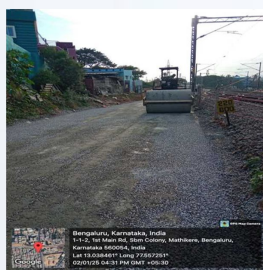
Blanket Top Layer Rolling Works
