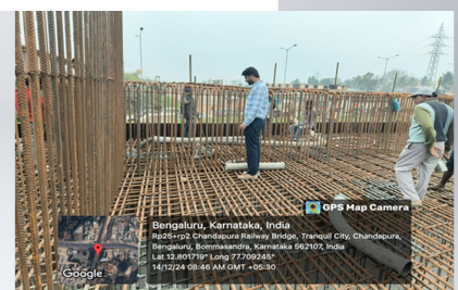
Br. No. 470 Pile cap of A1
