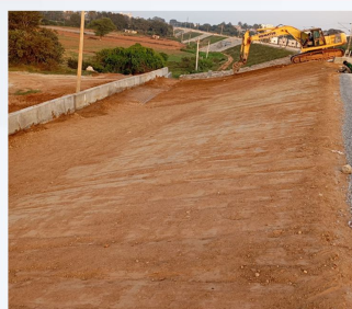
RUB Bridge. No. 424 / A Approach Earth work formation
