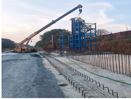
Raft Reinforcement works at Banasawadi, Fixing of Pier shutter for P7 and Portal Beam Crib staggering works is in progress for P2 & P3 at Kasturi Nagar of Mallige line.
