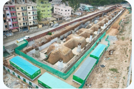
Bellandur Column works in progress
