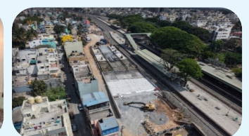
Ground Improvement work in progress at Banaswadi station
