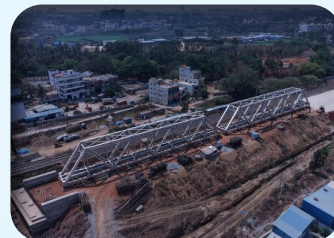
Aerial View of Assembled Girder at Major Bridge No 470
