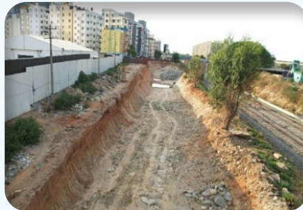
Earth excavation work in progress
