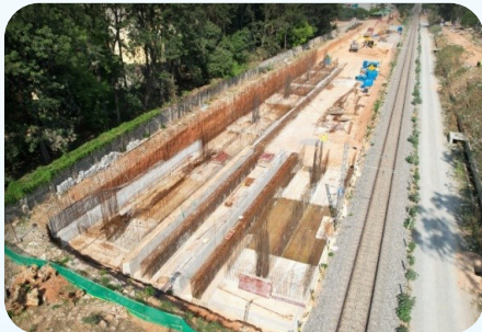
Raft Concrete works in progress
