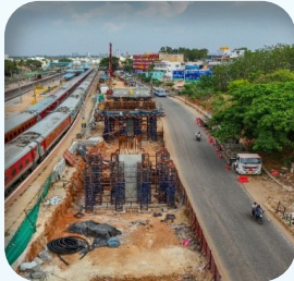
VIADUCT 625m. (From BAW toward SDVL)
