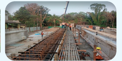
Casting in Progress for I Girder -1
