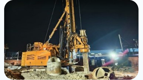
SP05 - 02 Piling work at Chikkabanavara station
