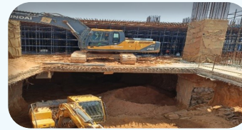
Yesvantapur station Grid no.6-8 Basement -01 Excavation work in progress
