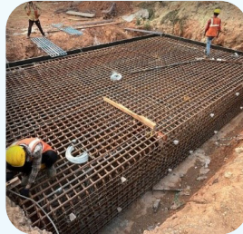
CP15 Pile cap reinforcement in progress for viaduct.
