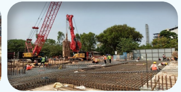
Ground slab b/w grid 10-11 Reinforcement fixing in progress at YPR Stn.
