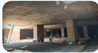
Raft reinforcement fixing for Slab for Grid no 2-3
