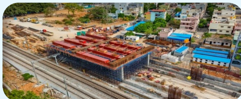
Concourse slab Reinforcement & shuttering work in progress
