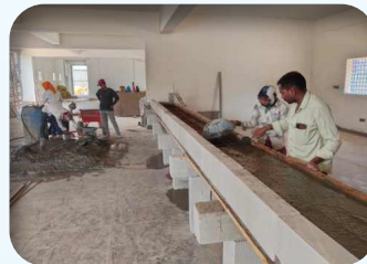
YPR, RRI Bldg. Parcel office Booking Counter
