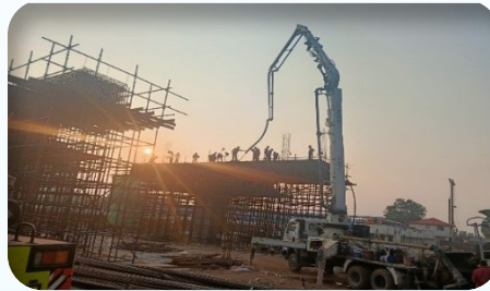
Pier arm SP03 Concrete pouring in progress
