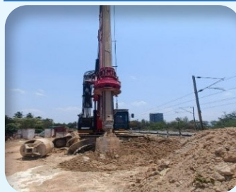
Piling works in progress.
