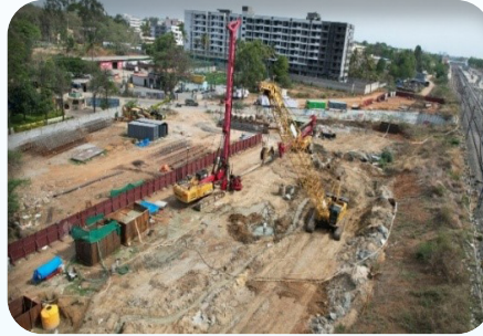
Piling works is in progress
