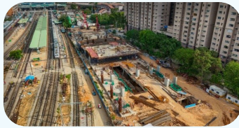
Ground slab -150 m and concourse slab 25 m casting completed
