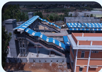
Aerial View of New Station Building and Foot-Over Bridge at Anekal Road Station
