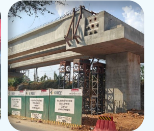
I Girder Erection 25m span of P19-P20 Chikkabanavara Viaduct
