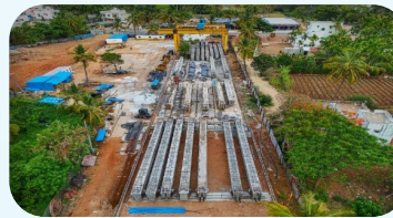
Casting in Progress for I Girder -1
