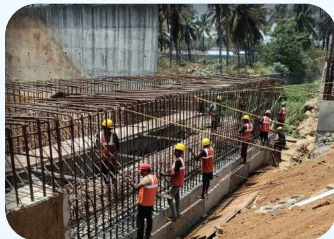
Br. No. 573; RCC box side wall Reinforcement & shuttering work
