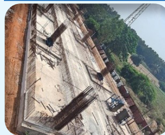
Raft Concrete works is in progress
