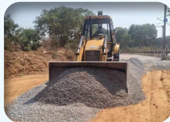
Railway formation Blanketing works in progress
