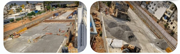
Raft concrete done at Hebbal Station GSB filling work in progress.
