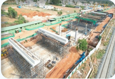
Portal beam work is in progress
