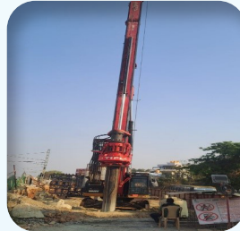
Piling in progress for PP4
