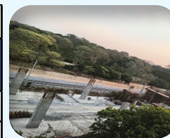
Portal beams P2 & P3 concrete completed
