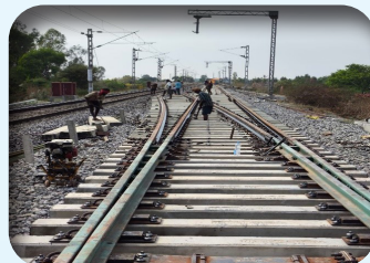
Track linking works between Maranayakkanahalli and Hosur Section
