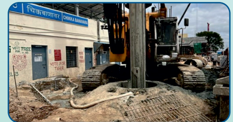
SP-06 RHS /03 pile boring
