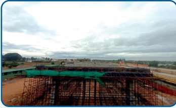
Portal Beam work in Progress
