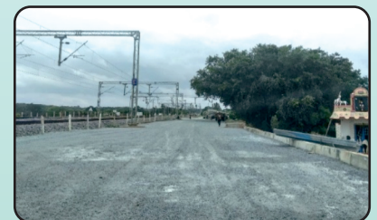
Blanketing work at KM 166
