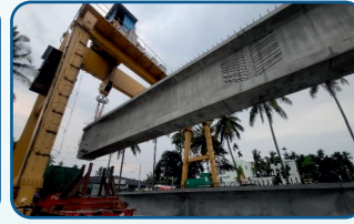
I-Girder Dispatched from Casting Yard
