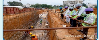
Retaining wall works
