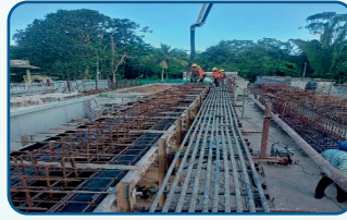
I Girder P9-P10 G4 Concrete pouring started
