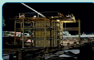
P 12 Pier concrete
