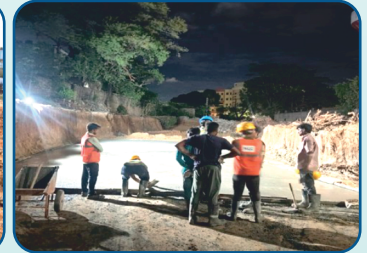
Station PCC in progress
