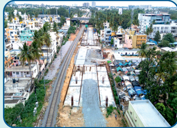
Aerial View of hebbal station
