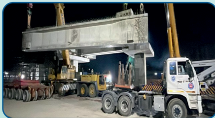
Grid 2-3 G3 I girder erection
