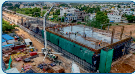
Concourse slab concreting work in progress b/w grid 11-13
