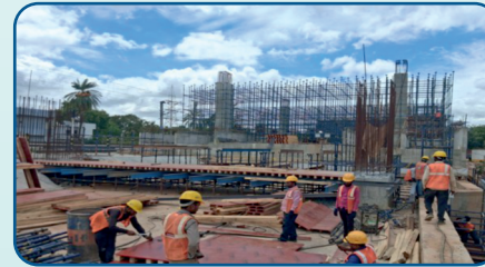
MYD portal beam staging and shuttering WIP B/w Grid 05-08
