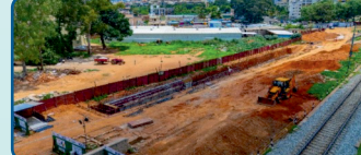
Retaining wall works
