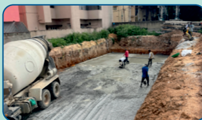
BAND RRI Building foundation PCC/Plaster work
