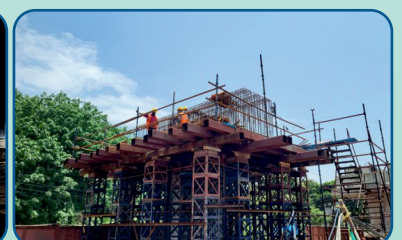
Reinforcement tying work for P7 Pier cap
