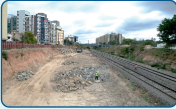
Raft Excavation works
