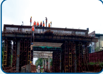
Portal beam Reinforcement bending work in progress.
