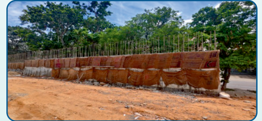
ERS concrete work of 1.2m lift height in progress.
