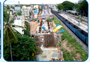
Aerial View of Banaswadi station
