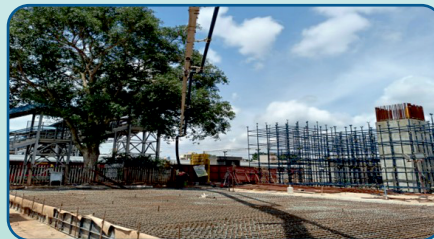
Grid 7-8 Raft concrete pouring
