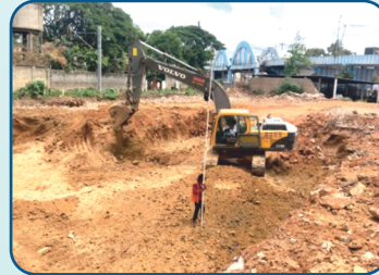
Station raft excavation
