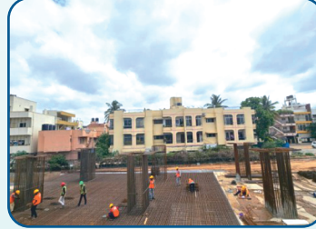
Basement Rebar work in Progress
