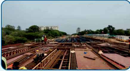
CCL & Portal beam reinforcement tying WIP at Grid no. 1-3
