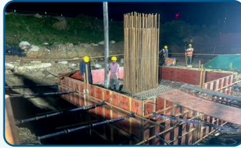
Pile cap concrete in progress
