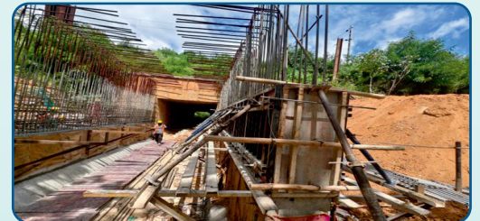
Sacrificial wall 1.2 Mts height formwork in progress.
