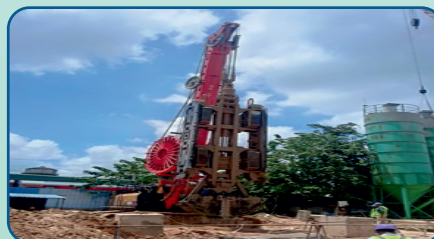
Barrette C-76 panel Grabbing & cage lowering WIP
