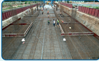
Raft reinforcement work
