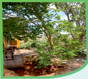
Excavation of Soil before tree uprooting
