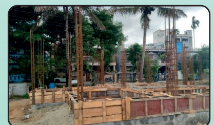
S&T Building at Hosur Yard
