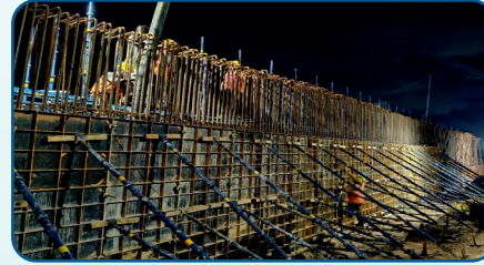
Retaining wall 2nd lift, Grid 05 to 06 Concrete work in progress
