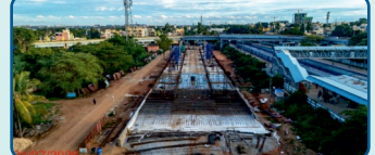
Raft Concrete works is in progress
