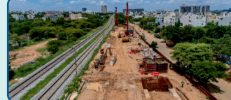
Pile reinforcement cage lowering
