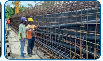
Reinforcement and profiling checked for girder G2, span P7-P8
