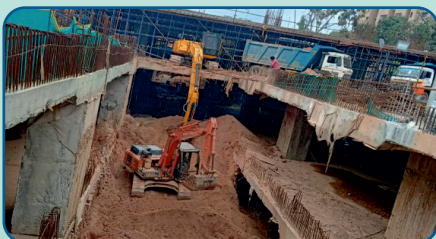
Basement-02 Grid 03-04 excavation work
