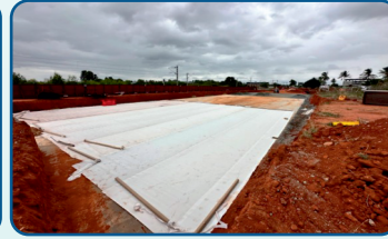
Water proofing works in progress
