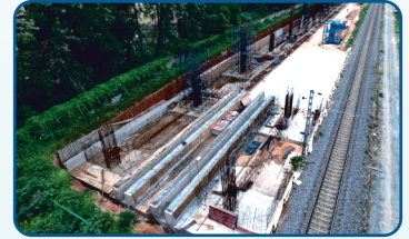
Kaggadasapura Station view
