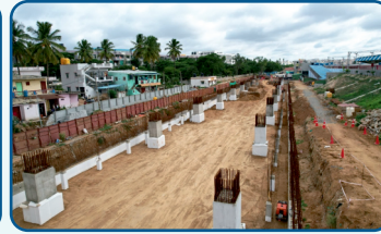
Bellandur Station view
