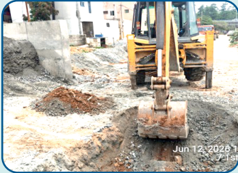
Retaining wall excavation
