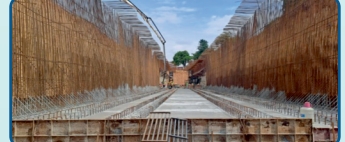
Staging and Reinforcement works for top slab
