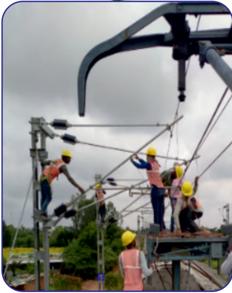
Tower Car checking and IOL (Insulated overlap) creation: As a part of doubling works IOL creation work is completed at Maranayakanahalli Yards.
