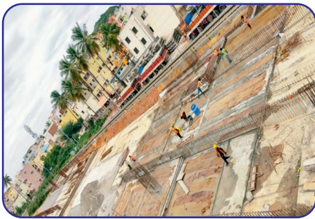
Raft concreting completed
