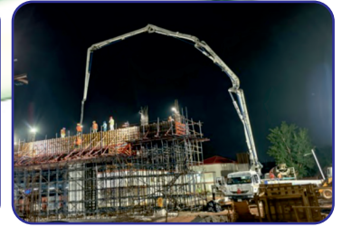
SP05 pier arm concreting is in progress
