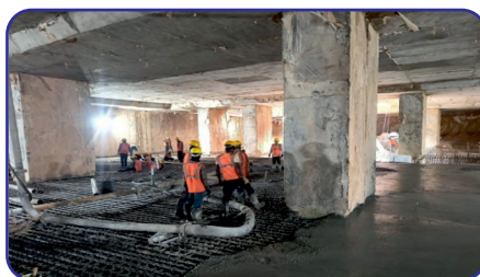
Structure Id: Basement 2 Grid 6-7 Concrete Pouring WIP
