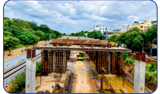
Portal beams P9,10,12,13 concrete done at Kasturinagar station
