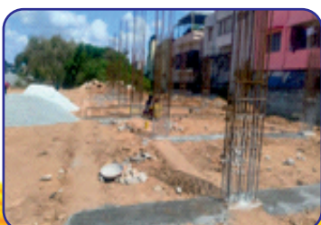
Banaswadi RRI Building's Plinth Beam work
