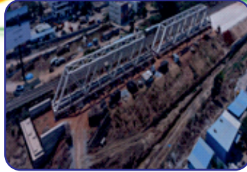
Br. No. 470: Both Girder assembling
