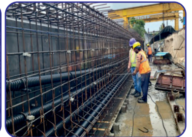
P13-P14 G1 I girder reinforcement and profiling work
