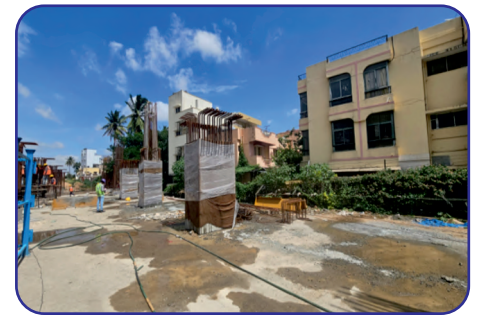
Banaswadi Station basement pier P4A,3A,C1,C1,5A curing
