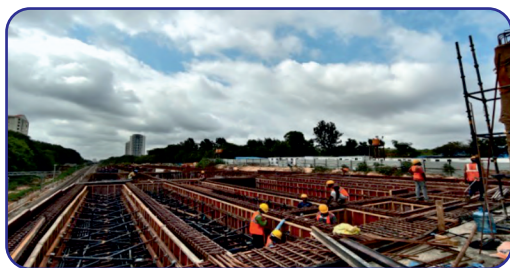
Grid 4-6 CCL beam shuttering WIP
