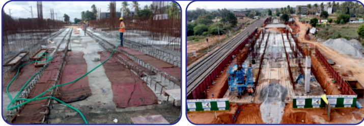
Singenaagrahara Station- Station Raft and Column work
