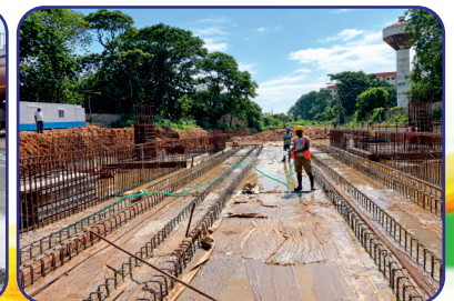
Raft Curing in progress
