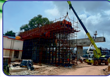
SP-07 pier arm shuttering WIP
