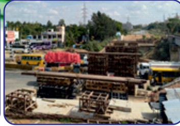
Br. No. 470: Temporary works for launching of girder
