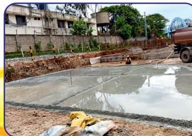
PCC curing in progress
