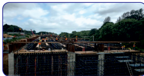
CCL SLAB REINFORCEMENT WIP GRID 11-13
