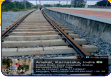
Track linking works in progress b/w MNKH-HSRA section
