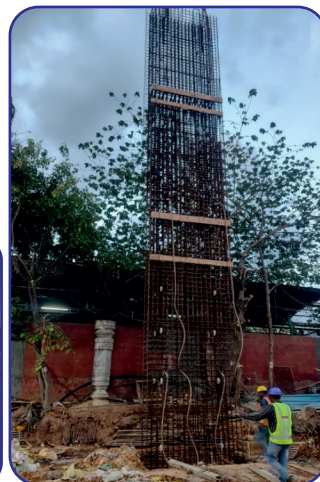
D-wall Panel ED 45 cage lowering work
