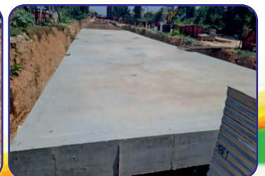
1st span of 45m, box top slab casting completed & 2nd span of 45m top slab ready for casting
