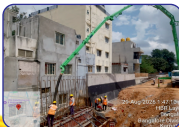
MIB 548 return wall 2nd lift wall concrete
