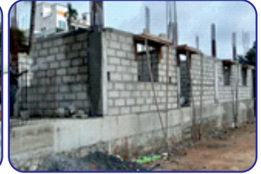
Construction of S&amp;T store cum office building at HSRA
