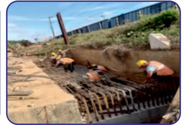
MIB 404 Top slab reinforcement works
