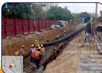
ERS wall raft concreting work
