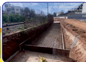
Sacrificial wall cast insitu raft reinforcement and formwork
