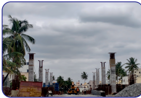
09no's Pier concrete is completed -P1A,6A,7A,7C,P8A,P8C
