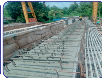
P13-P14 G14 I girder concrete
