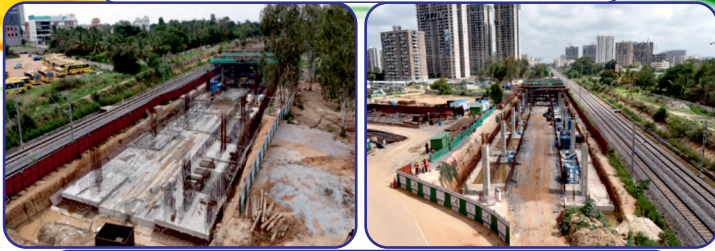
Singenaagrahara Station- Station Raft and Column work
