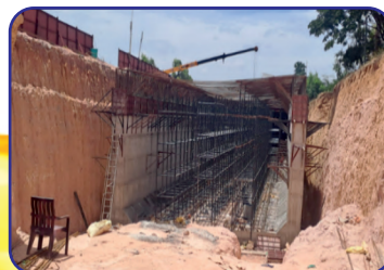
Staging for reinforcement works of top slab are in progress for 3rd span of 45m
