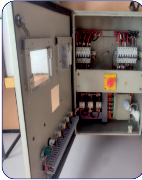
CLS erection work completed at LC 144A (Kanakanagar).
