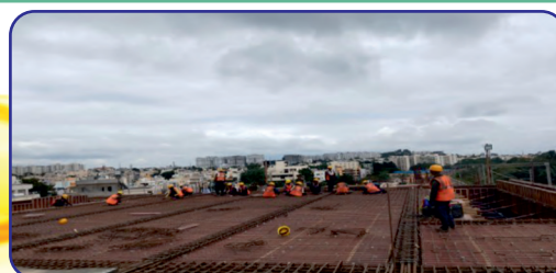
Grid 9-10 CCL slab reinforcement and shuttering work in progress
