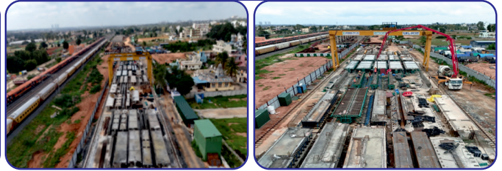
Casting Yard- Casting of Girder is in progress
