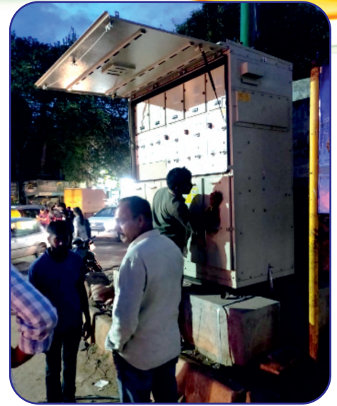
RMU (Ring Main Unit) erection completed in connection with utility shifting of Corridor-2 Section-3.
