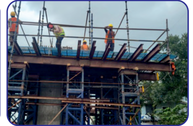
P13 pier cap bottom shutter alignment work
