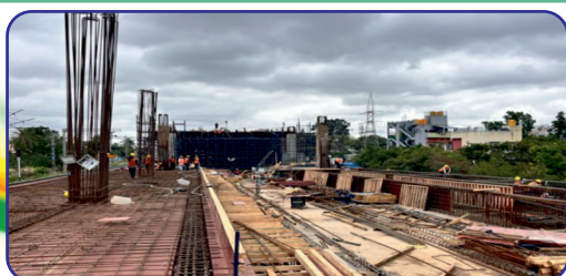
Grid-04 to 07 Platform level Slab shuttering and reinforcement fixing is in progress LHS and RHS
