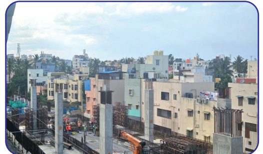
Banaswadi station work Progress
