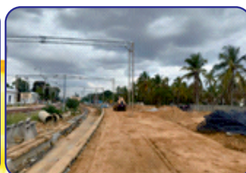
Hebbal Yard Platform's soil Compaction work
