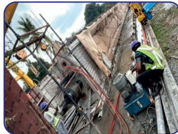
Post tensioning, I-Girder span P11-P12, G3 1st stage stressing
