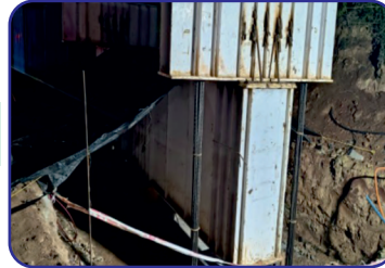
P18/1 static load test completed
